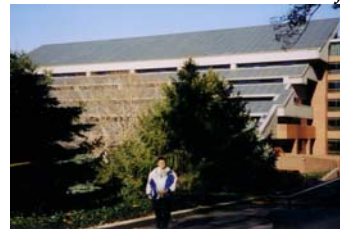
Installed Georgetown University 1984 in Washington, DC USA $65,000 BI-PV Solar Electric Yearly
