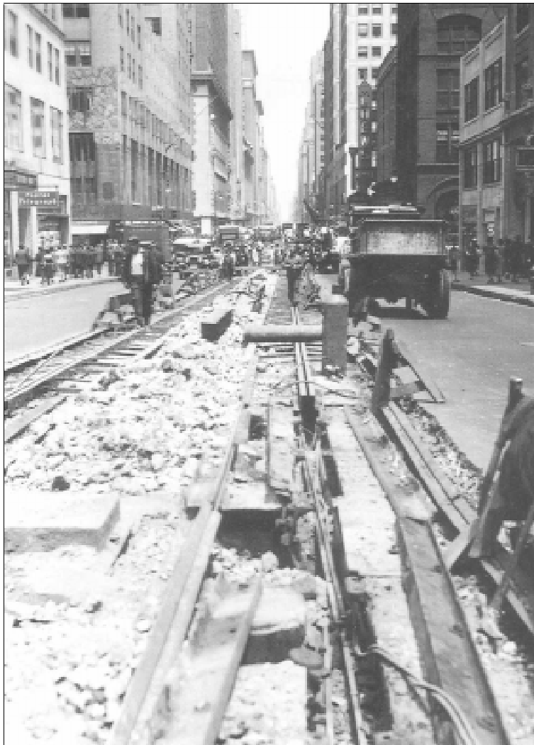
Picture 2.1-2: Tearing up Trolley Tracks
