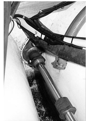
This bearing had to come out and be shimmed! Note: 1.5" Shaft
