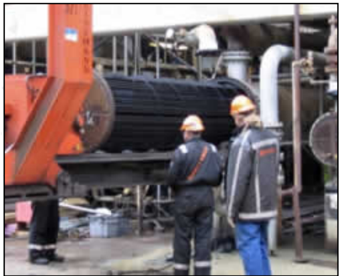
Fitting a Shell & Tube Heat Exchanger (photo courtesy of Paul Phillips)
