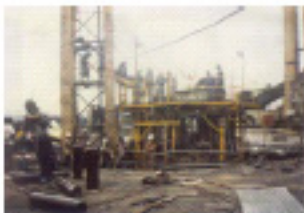
Taper Chimney assembly in progress
