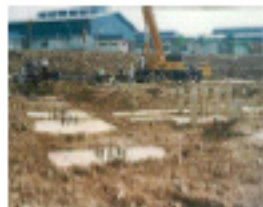
Civil works in progress at Tasek Cement, Malaysia
