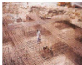
Reinforcement work in progress at Banjari Cement
