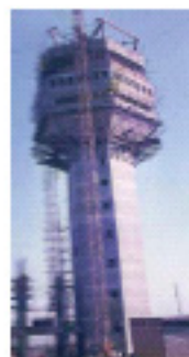
Air traffic control tower at Santa Cruz airport, Mumbai
