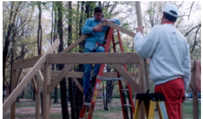
Master Roof Builders
