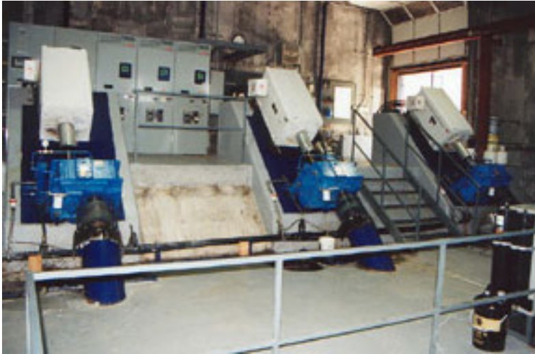
3 x 450 kW induction generator installation, Appleton Station, near Almonte Ontario.
