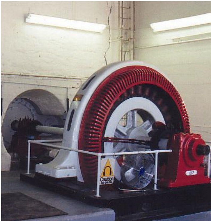
This Double Camelback Francis turbine/generator, built in 1903, is controlled by the TCM-30 at Galetta station near Arnprior
