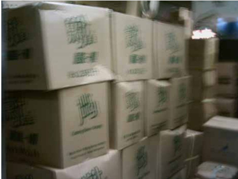
9. Paper boxes obstructing the corridor.
