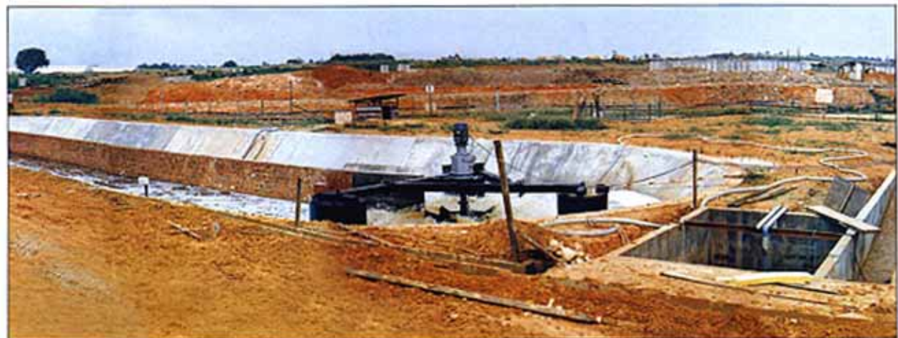
振顺乳牛农场 500头乳牛之氧化沟污水处理厂 Chin Soon Dairy 500 Dairy Cows & Milk Packaging Plant Oxidation Ditch WWTP
