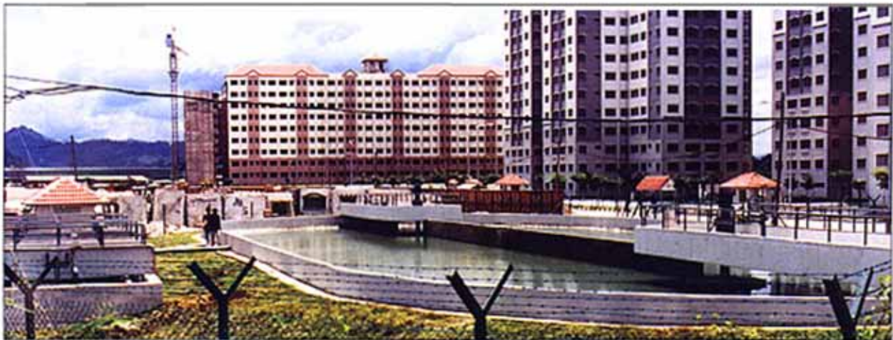
吉隆坡 Sunrise Mt Kiara 10000人口之氧化沟生活及处理厂座落于高密度住宅区 Sunrise Mt. Kiara, Kuala Lumpur 10,000 PE Oxidation Ditch S.T.P situated just next to the residential buildings
