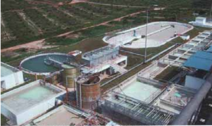
Oxidation Ditch Treatment for Rubber Latex Wastewater
