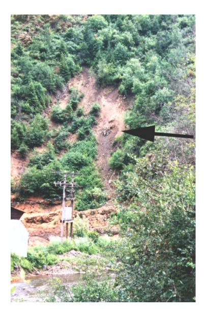
Figure 14: Photograph of landslide at site 27. Arrow indicates location of springs. *Landslide Type and Description*
