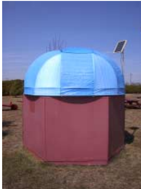
Solar Panel Installed
